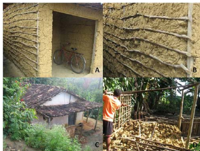
Fig. 4 Constructions with wood and mud in Três Ladeiras community (Pernambuco State, northeastern Brazil). (A, B) Arrangement of the wood in the construction; (C) painted wood and mud house; (D) dismantling process of a wood and mud construction.
